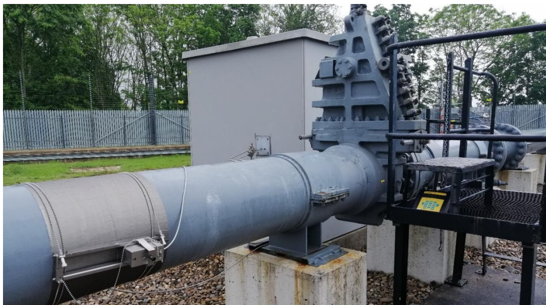
Figure 6: Clamp-on USM Installation
