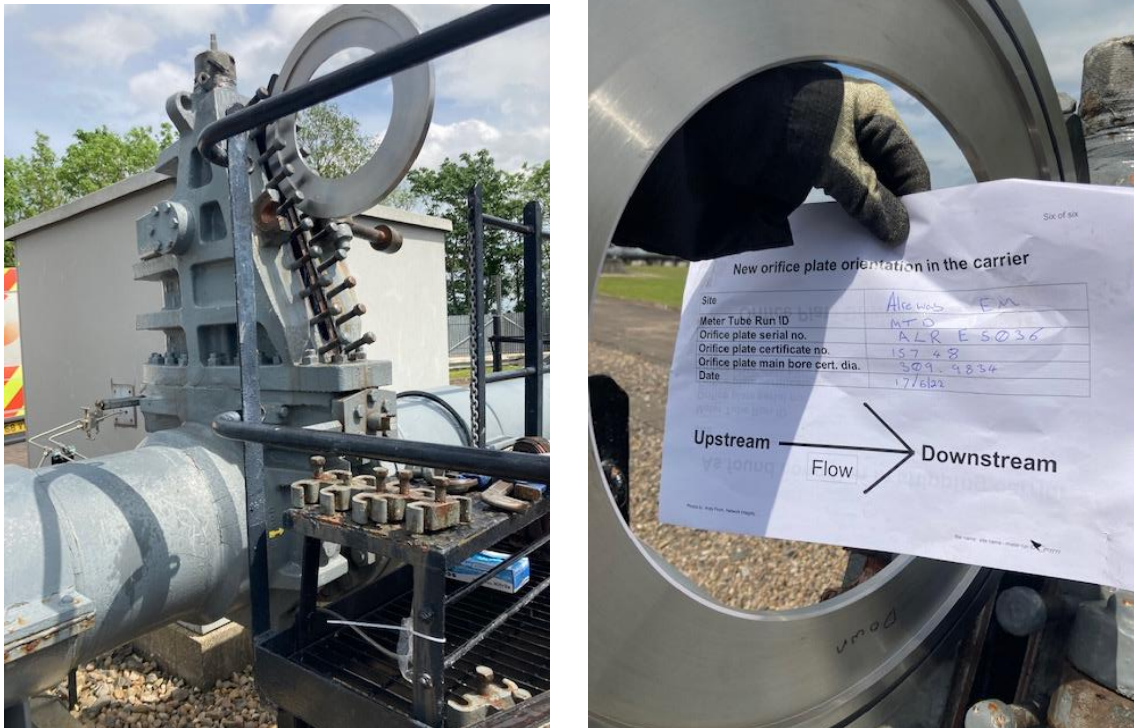
Figure 14: Flow Test 3 - Installation of plate 2 (ARLE5036)
