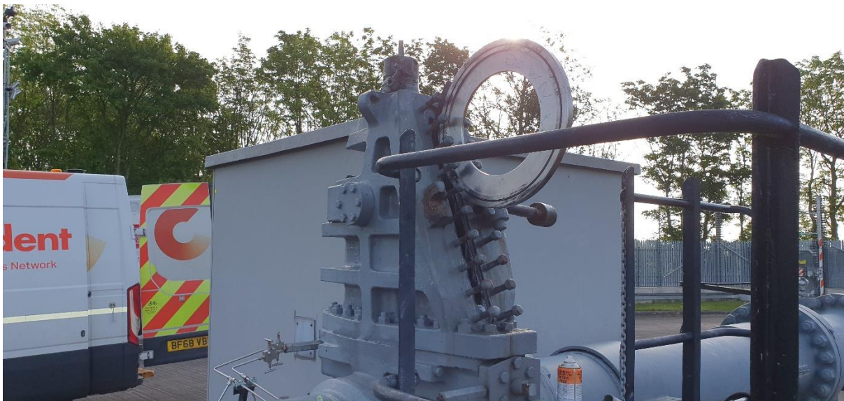
Figure 9: Flow Test 2 - Plate 1 (295/5) – Bevel Upstream
