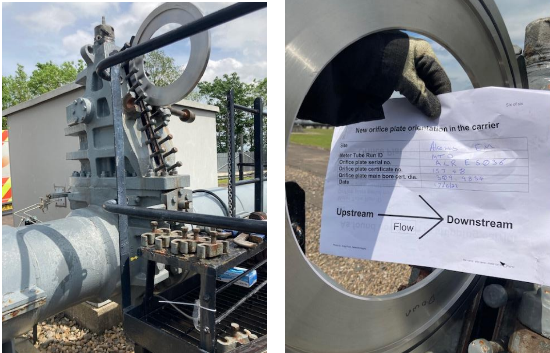
Figure 13: Flow Test 3 - Installation of plate 2 (ARLE5036)
