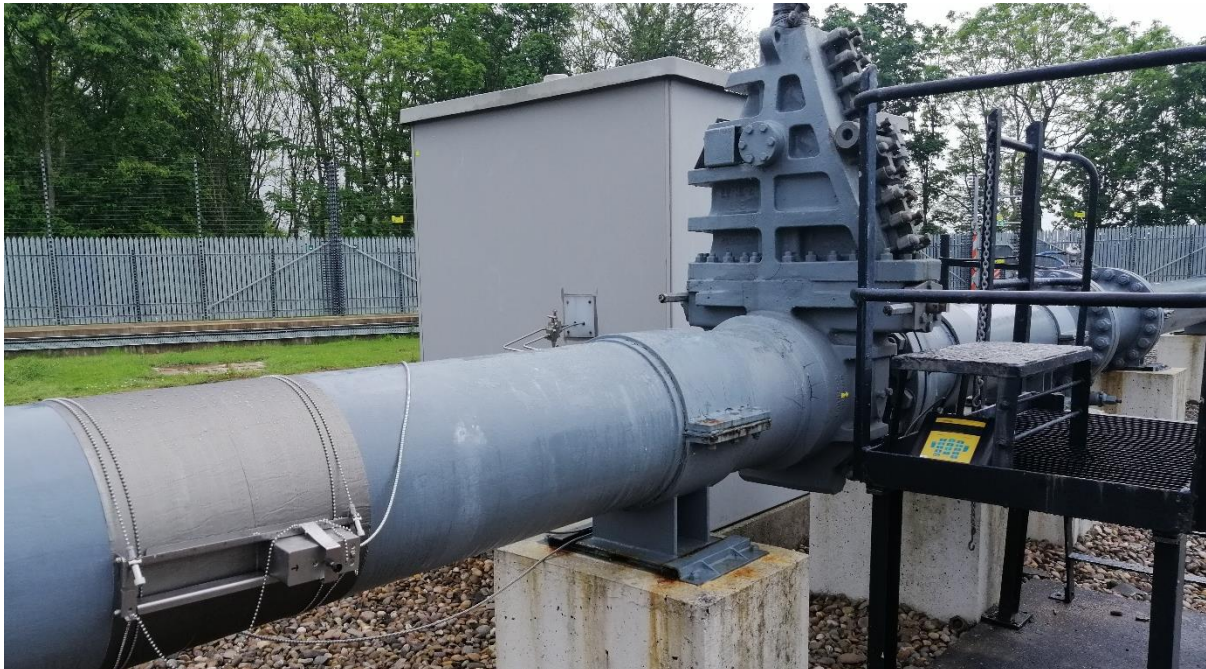
Figure 2: Clamp-on USM Installation
