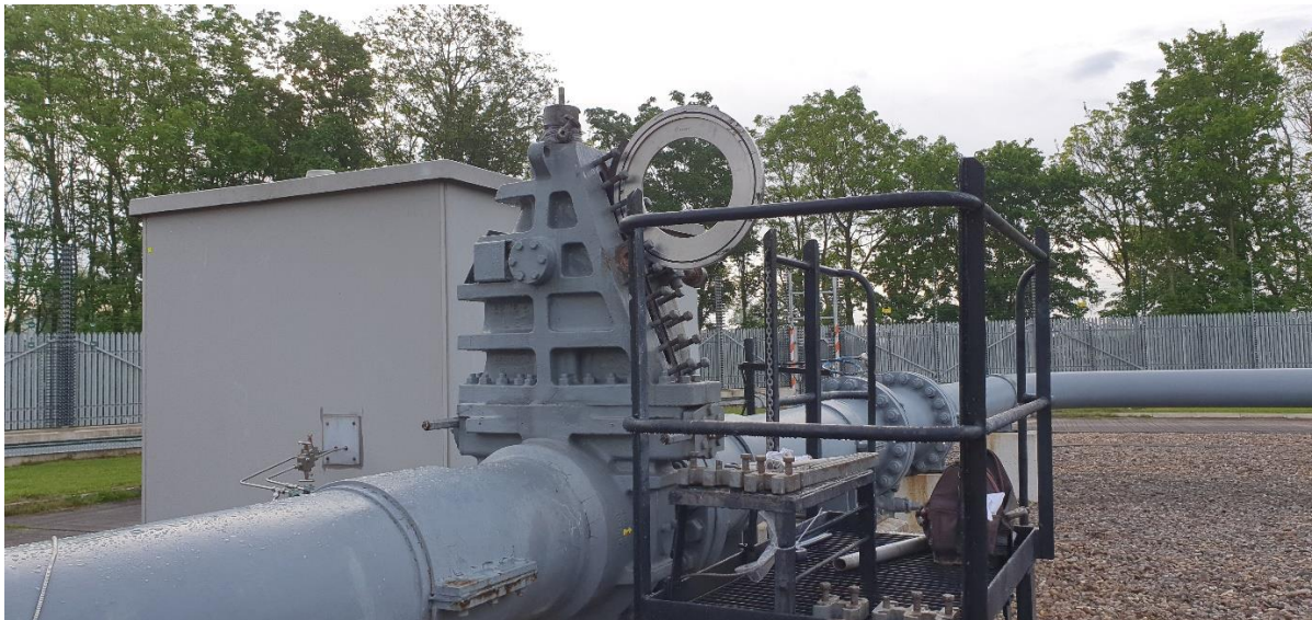
Figure 18: Flow Test 4 - Plate 2 (ARLE5036) – Bevel Upstream
