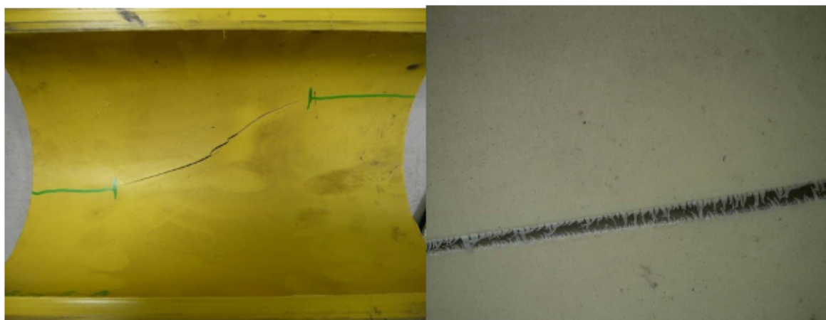
Figure 2: Example of SCG over 35 years in 1 st generation PE63 (Aldyl) pipe laid in rocky ground
