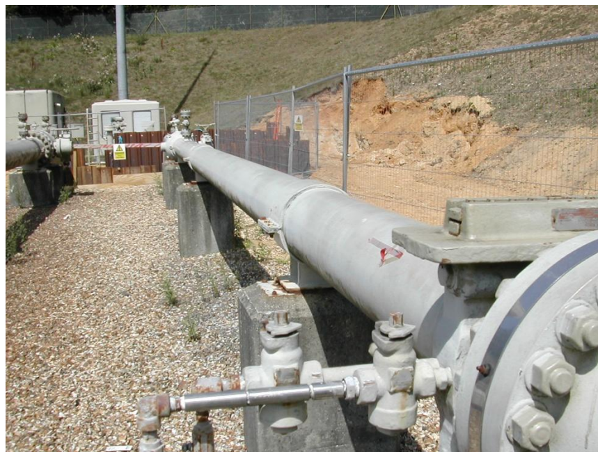
Figure 4.3 – Upstream Pipe Section
