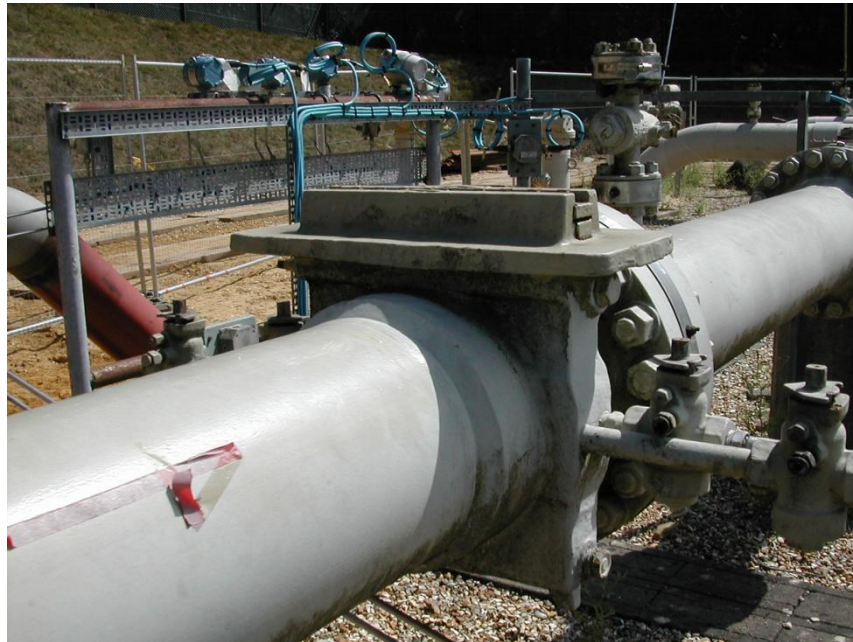
Figure 4.2 – Daniel Orifice Fitting
