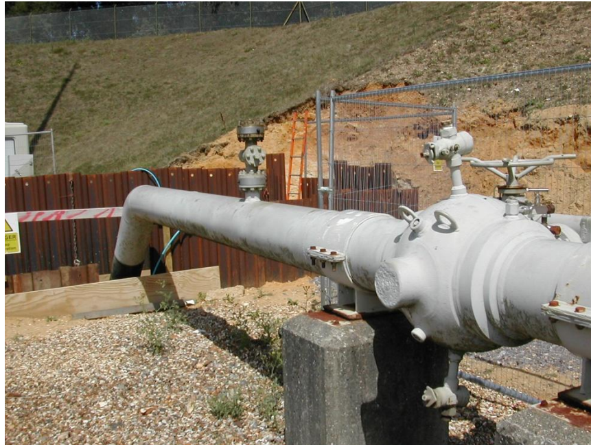
Figure 4.4 – Upstream Pipe Section Inlet
