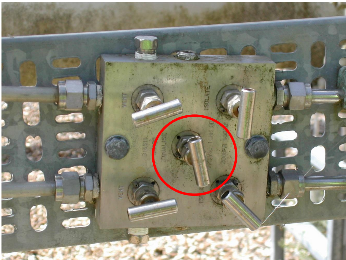
Figure 3.4 – Common \Delta P Isolation Manifold
