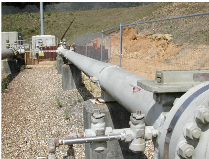
Figure 4.3 – Upstream Pipe Section
