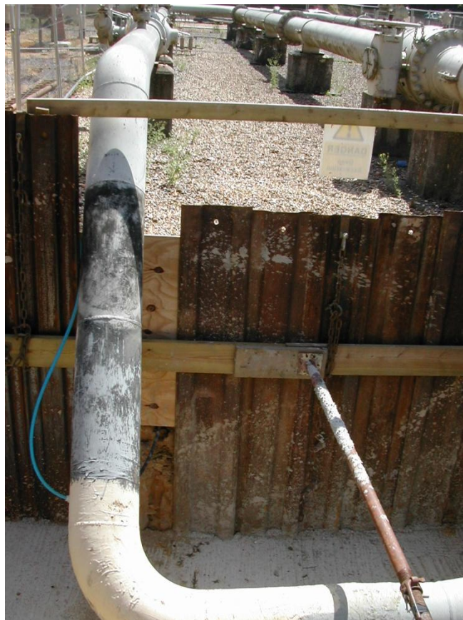
Figure 4.5 – Normally Buried Inlet Section
