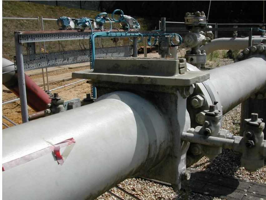
Figure 4.2 – Daniel Orifice Fitting
