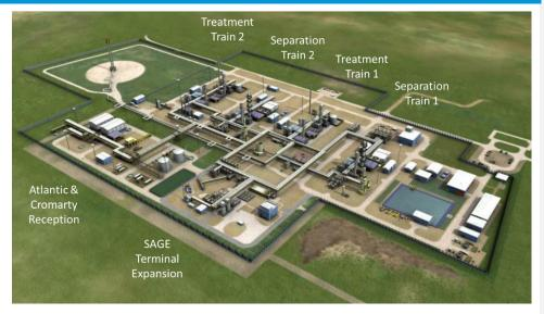
The original design of the SAGE facility included two identical amine absorption-based acid gas treatment trains each designed to remove around 1200 tonnes per day of  $CO_2$ . The acid gas stream was incinerated to oxidise  $H_2S$  and then vented to atmosphere. At design rates, each train consumes approximately 15 MW of fuel gas and 3 MW of electrical power.
