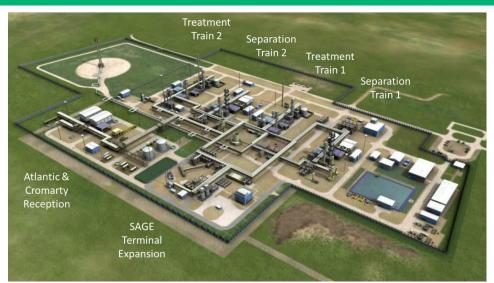
The original design of the SAGE facility included two identical amine absorption-based acid gas treatment trains each designed to remove around 1200 tonnes per day of CO<sub>2</sub>. The acid gas stream was incinerated to oxidise H<sub>2</sub>S and then vented to atmosphere. At design rates, each train consumes approximately 15 MW of fuel gas and 3 MW of electrical power.
