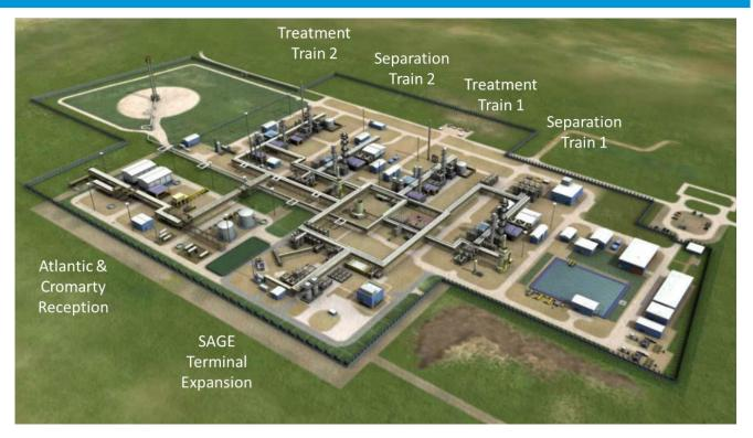
The original design of the SAGE facility included two identical amine absorption-based acid gas treatment trains each designed to remove around 1200 tonnes per day of  $CO_2$ . The acid gas stream was incinerated to oxidise H<sub>2</sub>S and then vented to atmosphere. At design rates, each train consumes approximately 15 MW of fuel gas and 3 MW of electrical power.
