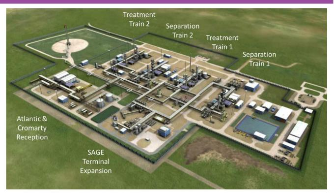
The original design of the SAGE facility included two identical amine absorption-based acid gas treatment trains each designed to remove around 1200 tonnes per day of CO<sub>2</sub>. The acid gas stream was incinerated to oxidise  $H_2S$  and then vented to atmosphere. At design rates, each train consumes approximately 15 MW of fuel gas and 3 MW of electrical power.
